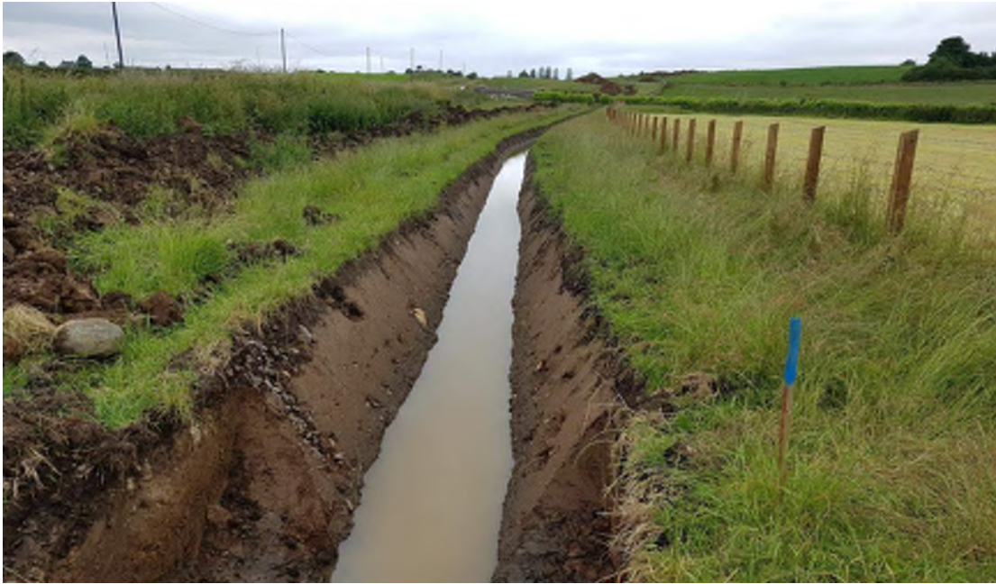
Plate 6.1 Example of cut-off ditch
