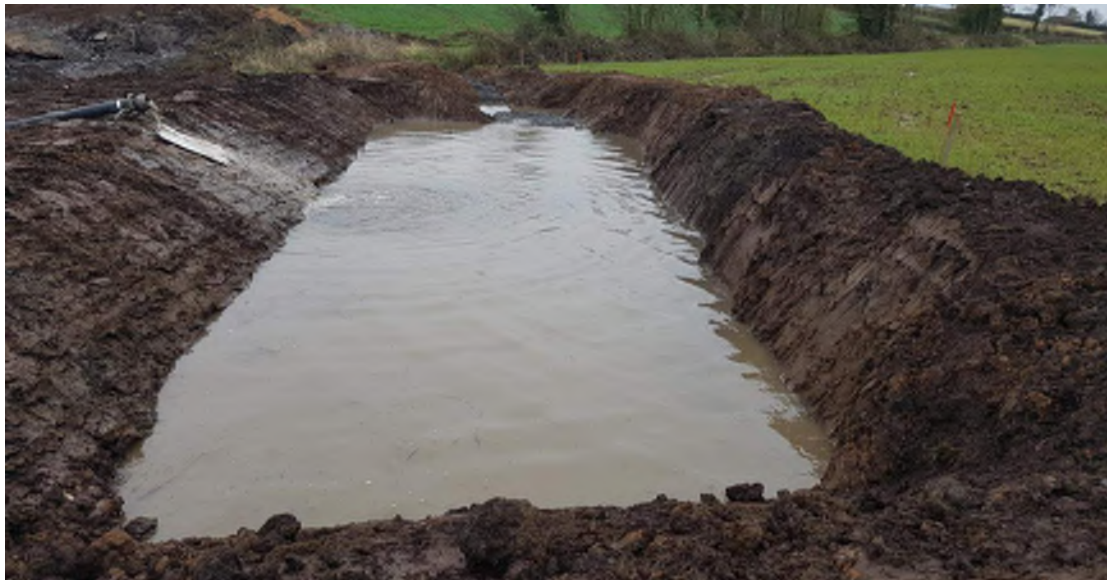
Plate 6.5 Typical temporary settlement pond / lagoon
