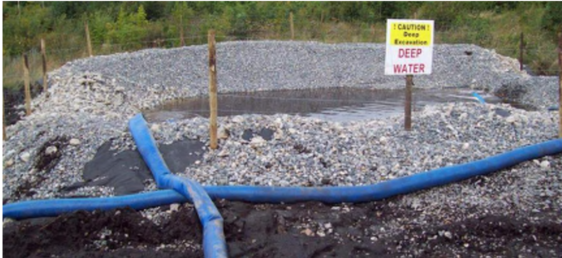
Plate 6.4 Typical temporary settlement pond / lagoon
