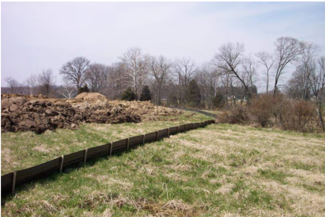
Plate 6.2 Typical silt fence usage
