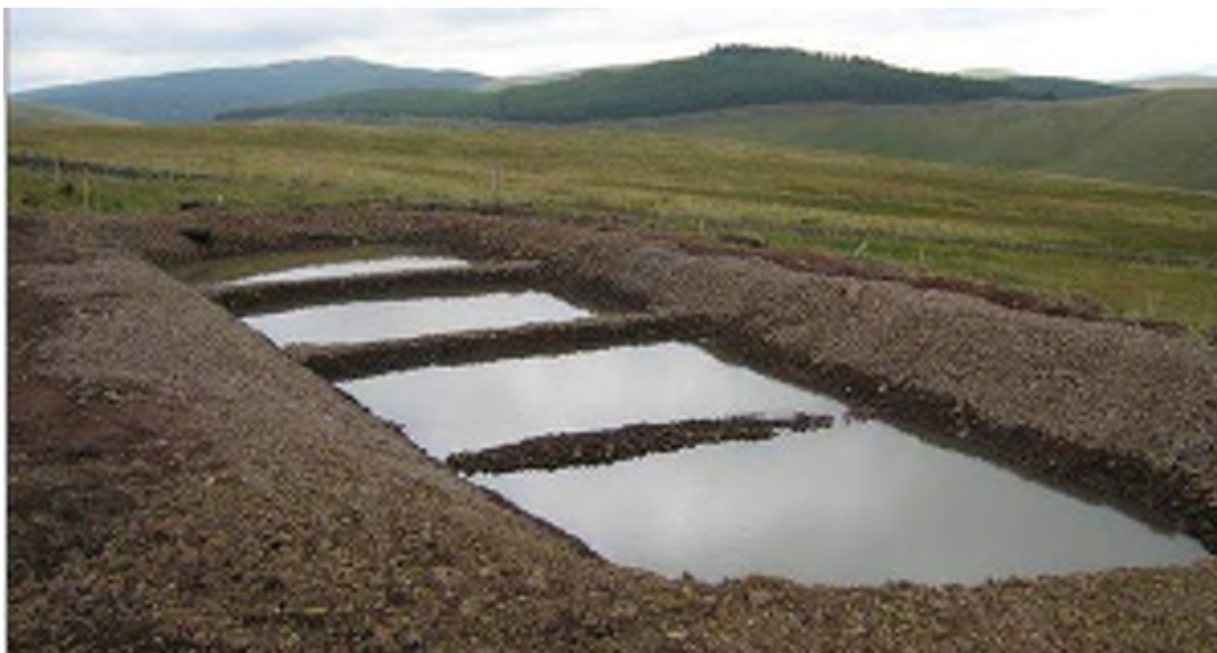
Plate 6.3 Typical temporary settlement pond / lagoon
